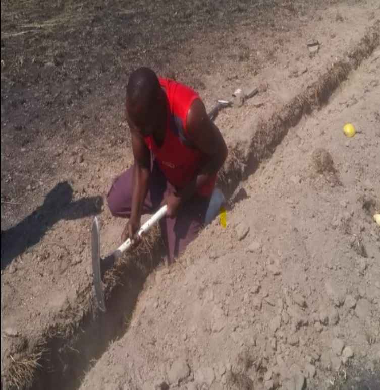
The villagers helped to dig the trenches.
